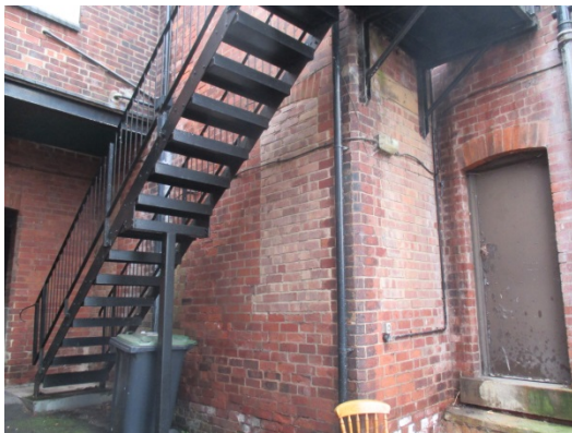
Rear of 250, former window openings
